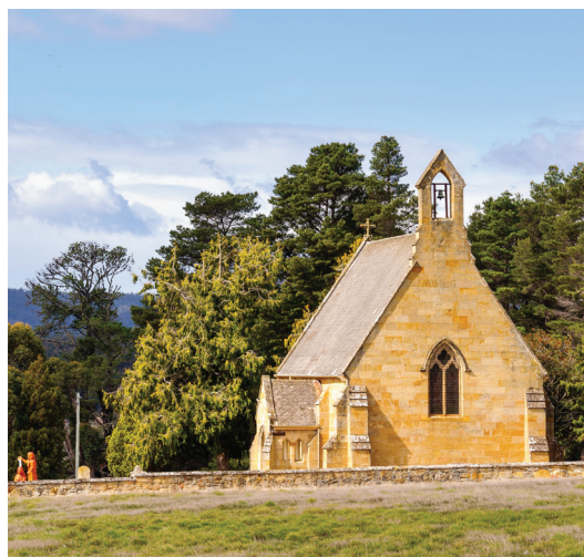
Buckland Church (ST)
