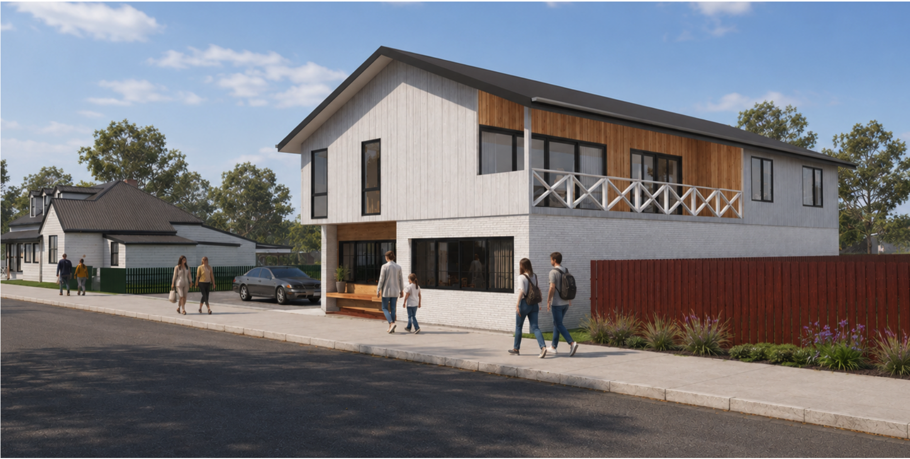
South West View
