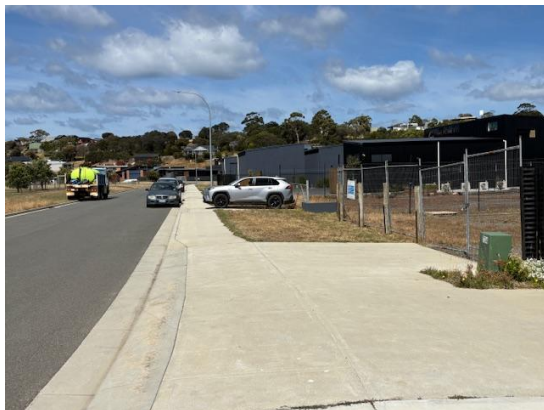
Figure 14– Side view of accesses to 70 & 72 Kunzea Circuit
